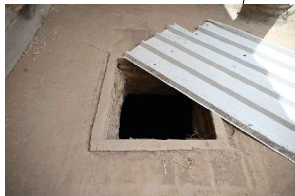
there is no protection bar for the holes shed to the basement
