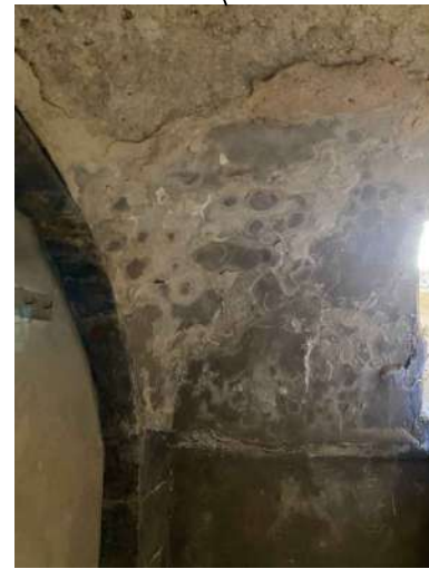
The high moisture of the basement cause erosion and salt to the concrete for walls and swelling for the material
