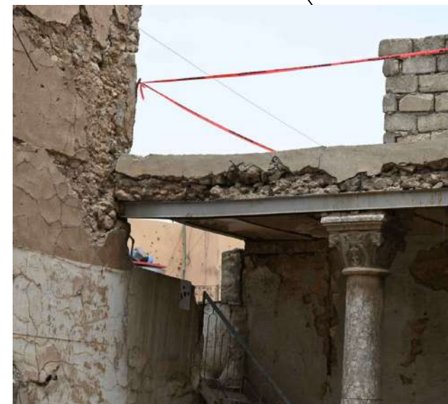
slab is dangerous and the c steel section was extended and caused a gap between 2 sections which allowed birds to build nests
