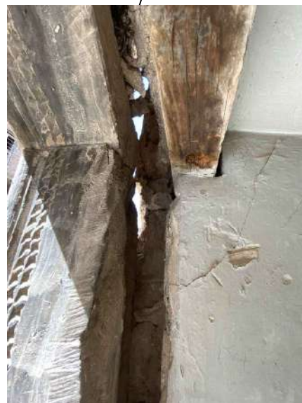
old gate prone to falling and need to support and bond to the wall
