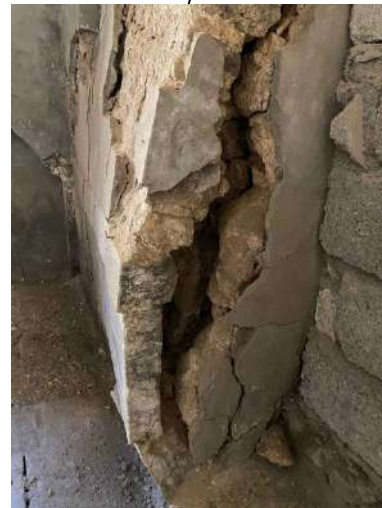
the wall in the kitchen basement swollen and prone to falling because of the explosion in the near area
