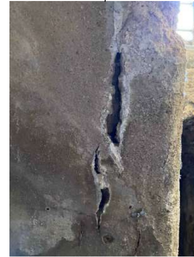
The high moisture of the basement cause erosion and salt to the concrete for walls and swelling for the material
