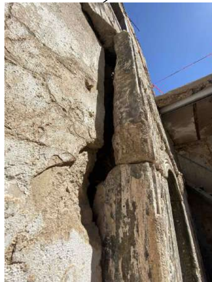
old gate prone to falling and need to support and bond to the wall
