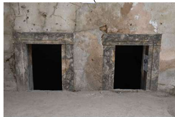
there is no protection bar for the holes shed to the basement
