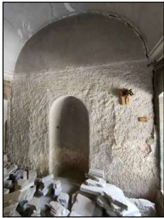
A wall with arches and deformed plaster
