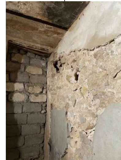
the wall in the kitchen basement swollen and prone to falling because of the explosion in the near area
