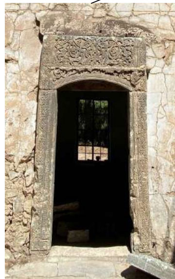
old gate prone to falling and need to support and bond to the wall
