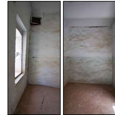
this photo shows a crack between the interior walls and exterior walls due to weak connection between them and this crack is obviously noticed inside every room
