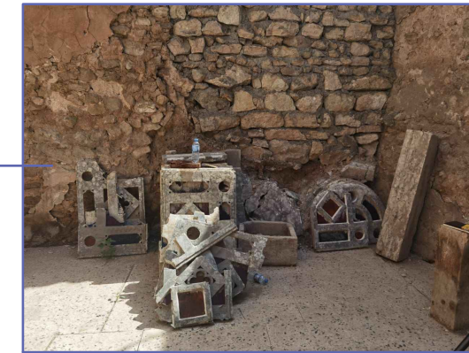
Antique windows in the courtyard were brought from another place part of the wall was reconstructed after destruction with cement and stone
