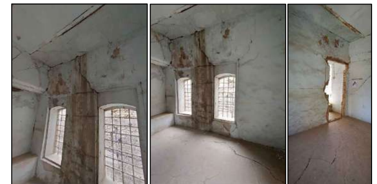
this wall is suffering from moisture problems it could be a leakage from the drainage pipe
