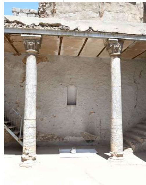
The old columns in the main courtyard which is reuse from another church
